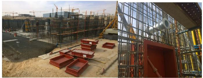
Picture 4&5: Temet blast door and wall sleeve installations in the construction site
